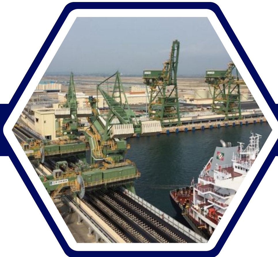
• TERMINAL O&M AND STEVEDORING SERVICES
